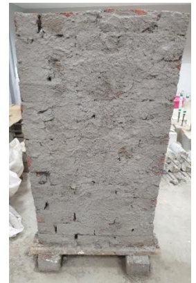
b- Application of splash cementitious coat.
