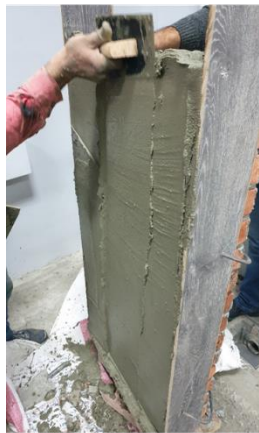
e - Final layer of PM mortar is applied.
