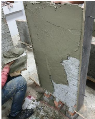
c-Apply first layer of PM mortar.
